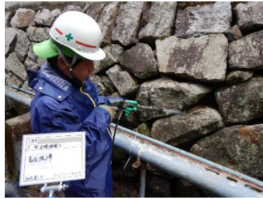
⑤目地汚れ高圧水洗浄
